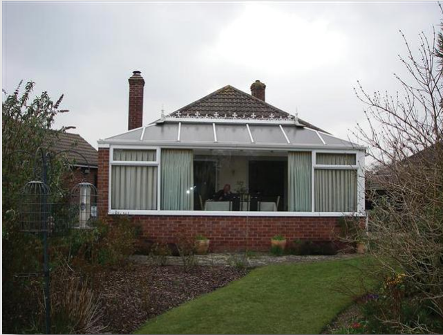
EXISTING CONSERVATORY TO REAR OF PROPERTY
