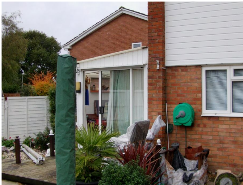
Current Conservatory, to be demolished, 2 Hemlock Road in Background, the front of the new build will be slightly to the left of the hose reel.
