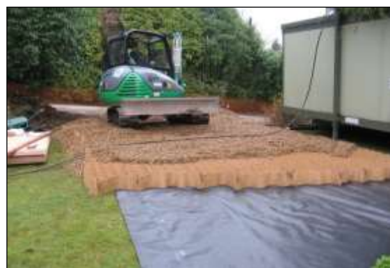
Photo 25: The stone-filled cells spread the load of traffic and the geotextile membrane on the ground prevents migration of the stone into the soil profile.
