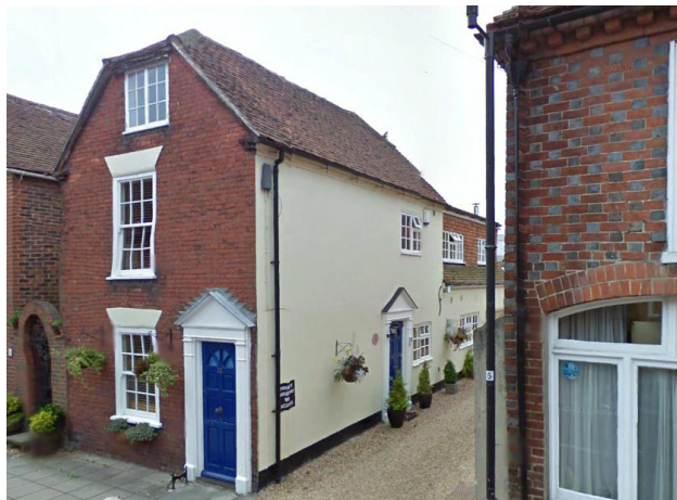
Site Photo - South Street
