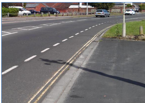
Photograph 4 Carriageway margin on Selsmore Rd.
