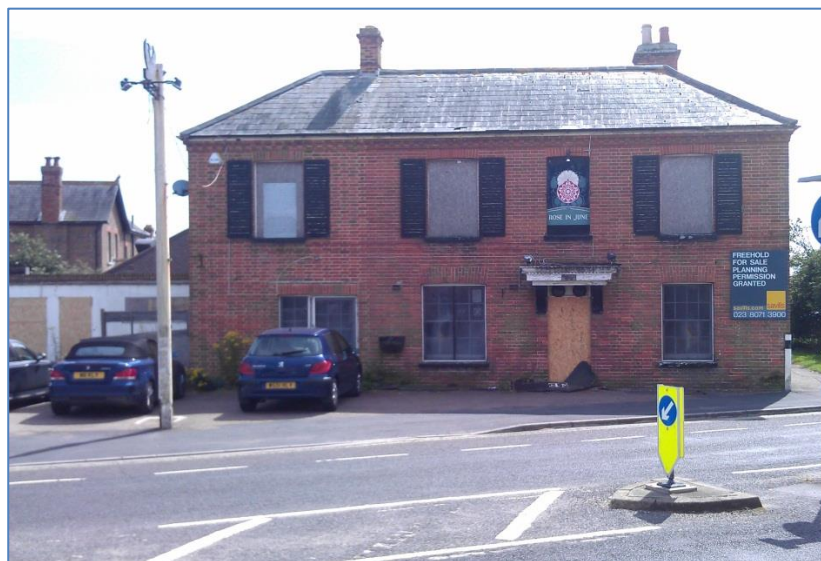
Photograph 1 Existing Development: The Rose in June
