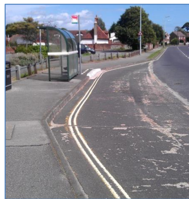
Photograph 6 Vehicle Crossover for Servicing
