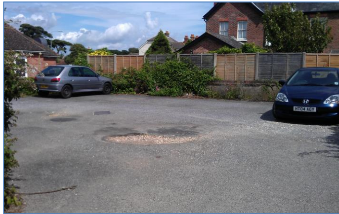
Photograph 2 Rear Staff Car Park
