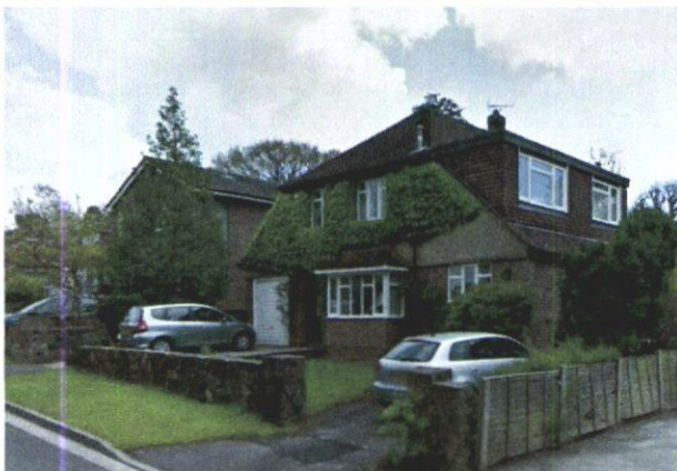
FRONT SIDE VIEW (NORTH WEST)
