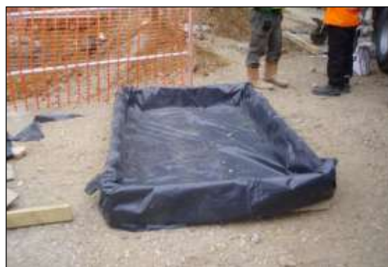
Photo 47: Soil bunding or a supporting framework covered in heavy-duty plastic sheeting is essential where there is a risk of spillages contaminating RPAs. This specifically applies to cement mixing areas and vehicle washing facilities.
