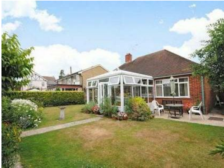
REAR VIEW (SOUTH EAST)
