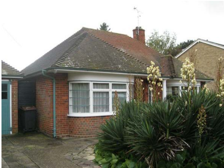
FRONT VIEW (NORTH EAST)
