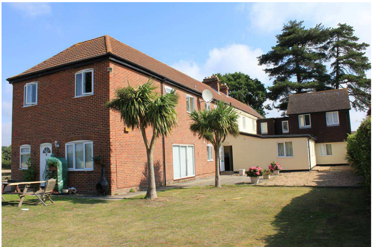
Photo 8 – View looking north-east towards the rear of the hotel with recent extension right of centre.
