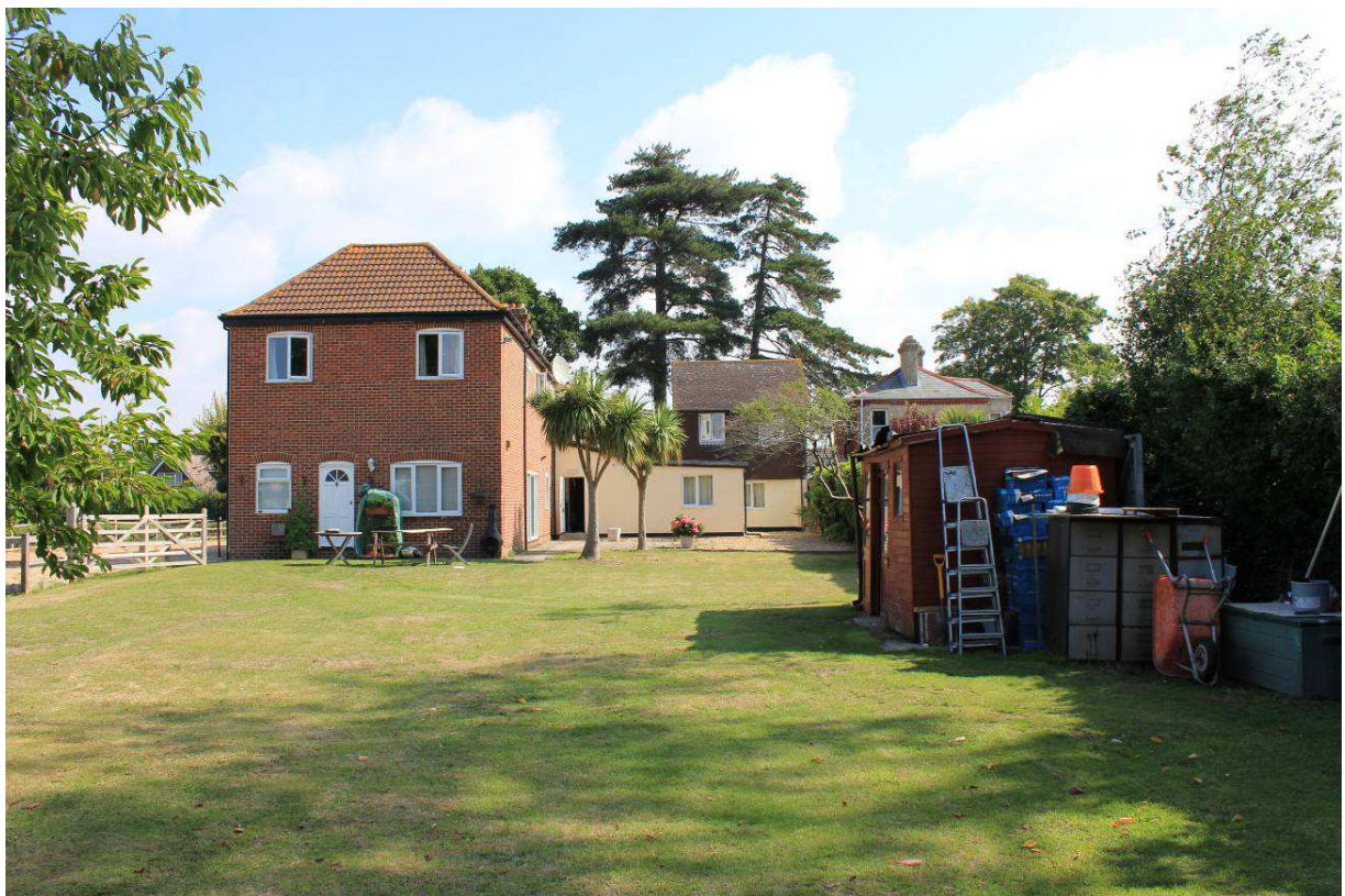
Photo 6 – View looking east with the south-east boundary to No. 75 on the right.
