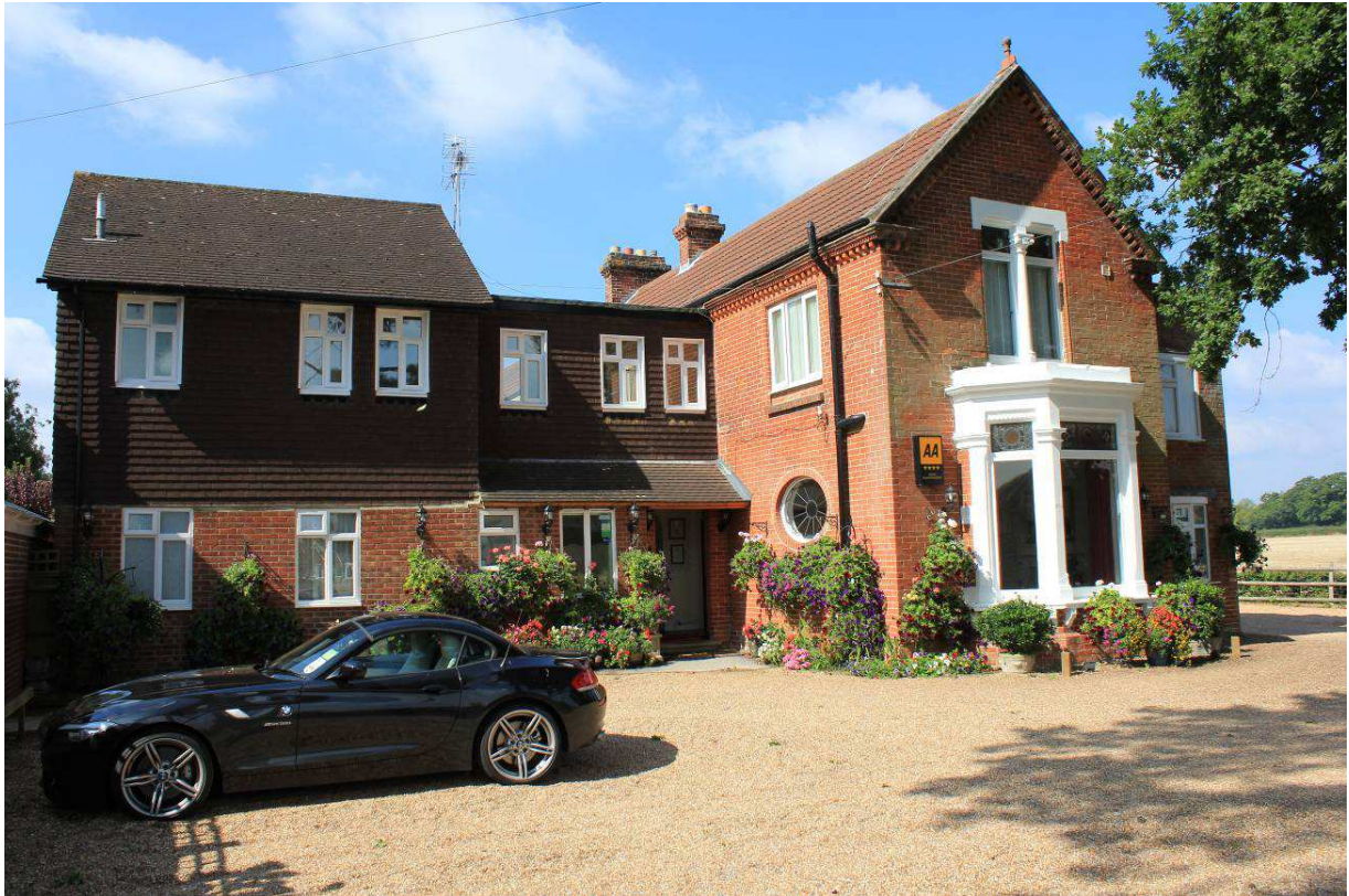
Photo 1 –Main entrance to hotel and north-east elevation..
