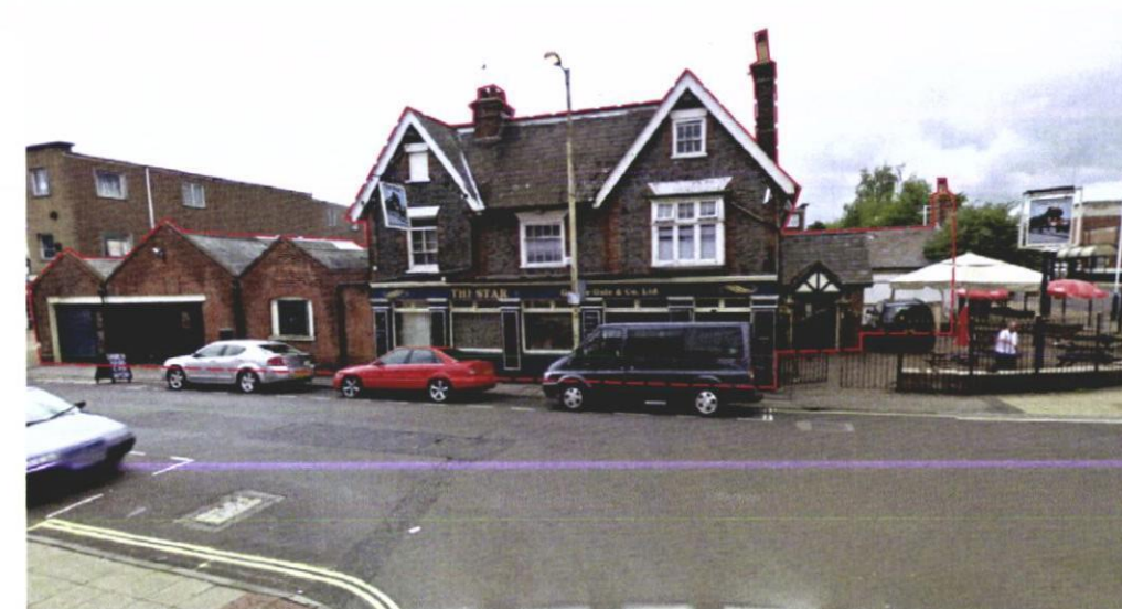
View of the existing Star Public House and gardens viewed from Waterloo Road
