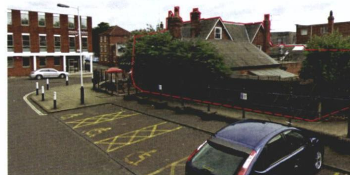
Existing Star Public House viewed from the Railway
