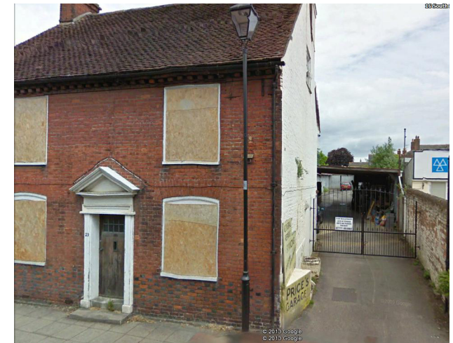
Site Photo - 23 South Street Narrow entrance leading to the rear development site. Refurbishment of no. 23 including the new extension has been completed.
