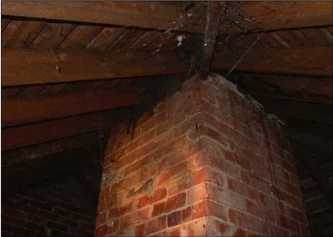
Photo14: Internal Chimney Structure
