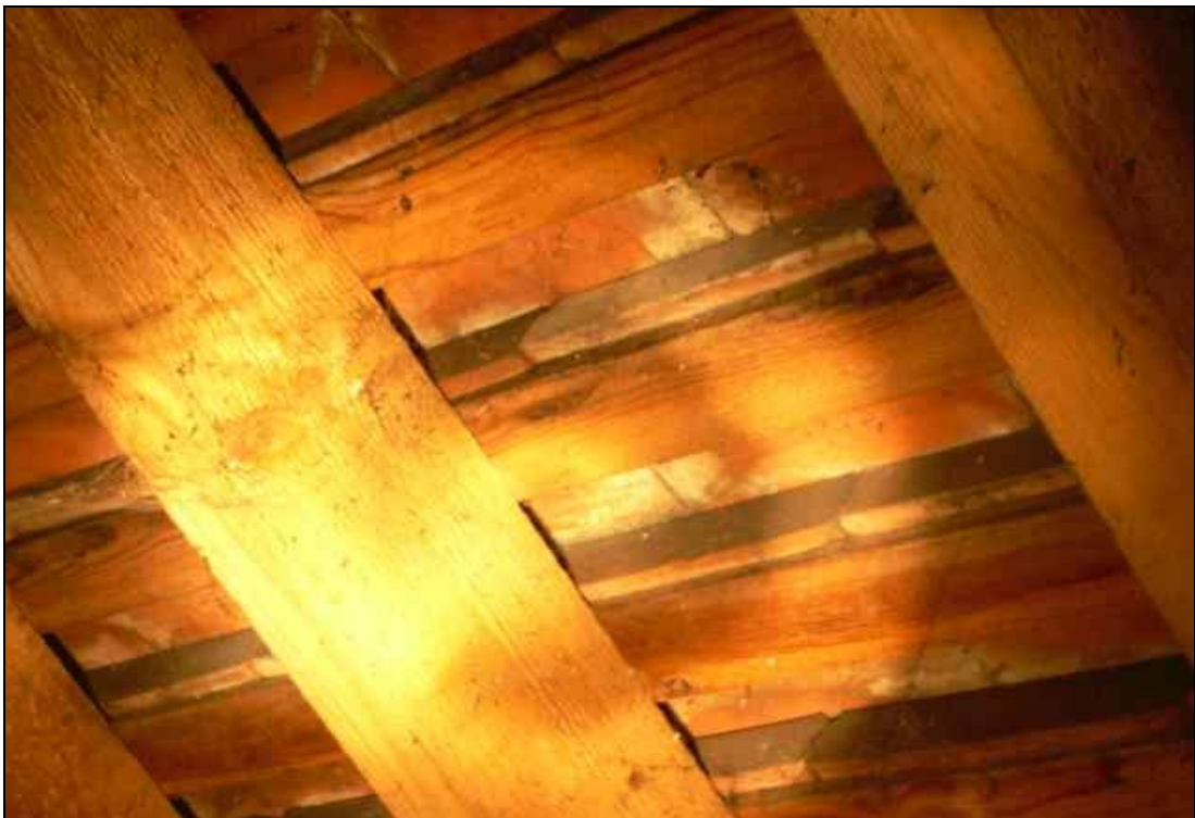
Photo15 The internal roof structure was fully accessible with the roof void. The roof tiles are hung direct onto the timber structure with no felt or roofing membrane resulting in a cold and drafty loft space.
