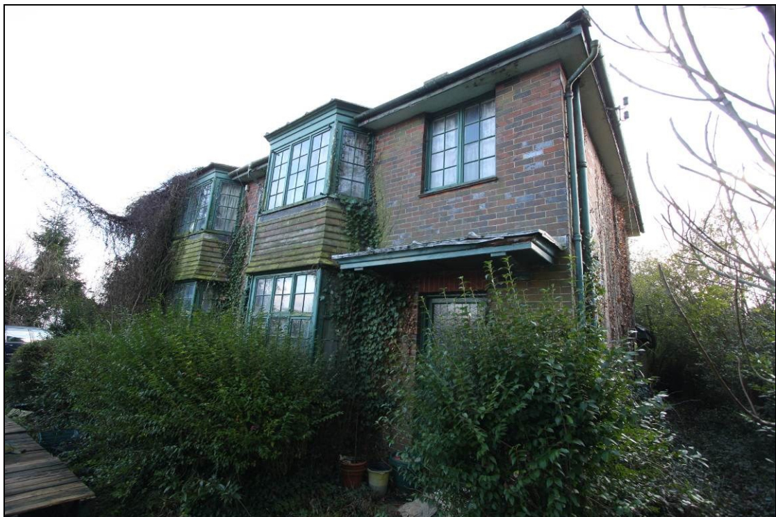
Photo 11 Manor Farm House is 2 semi-detached houses
