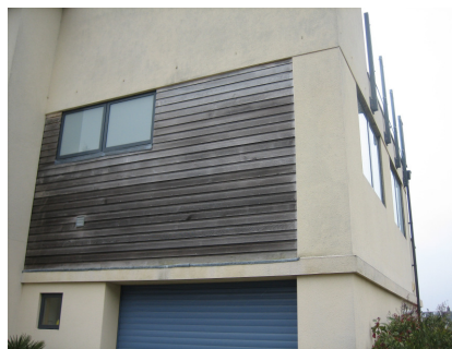
Fig. 9 – Weatherboarded feature to facade
