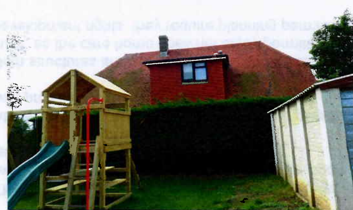
Dormer window to 26 Alexandra Avenue and play equipment
