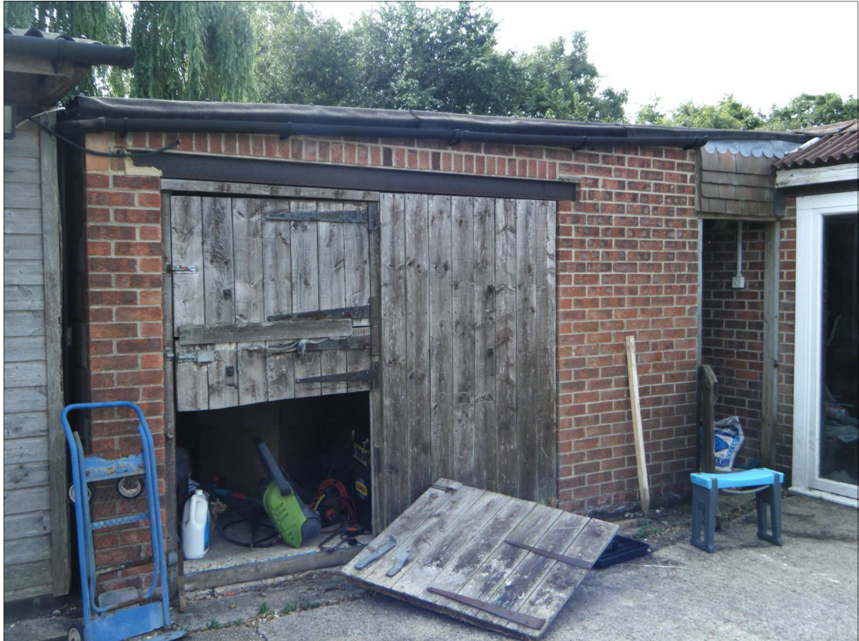
One of the outbuildings to be demolished
