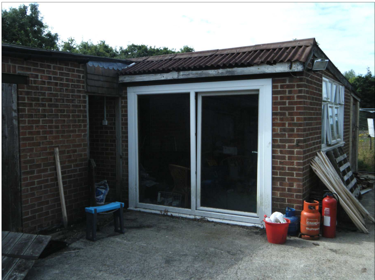
One of the outbuildings to be demolished
