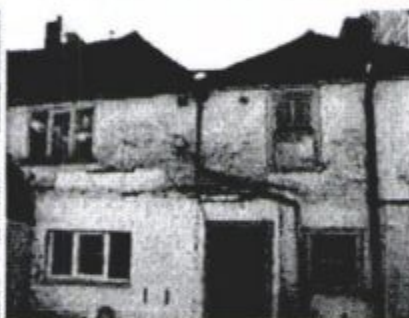
Figure 3 Northern Elevation of Building
