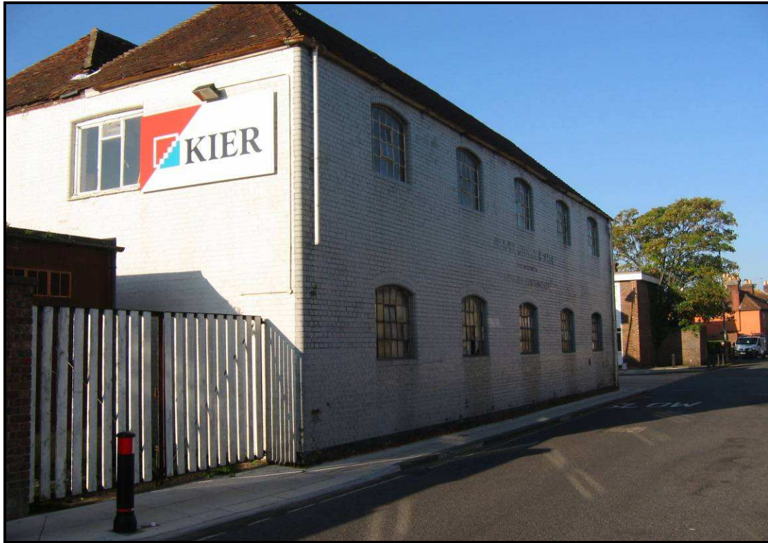
Existing Joinery Building
