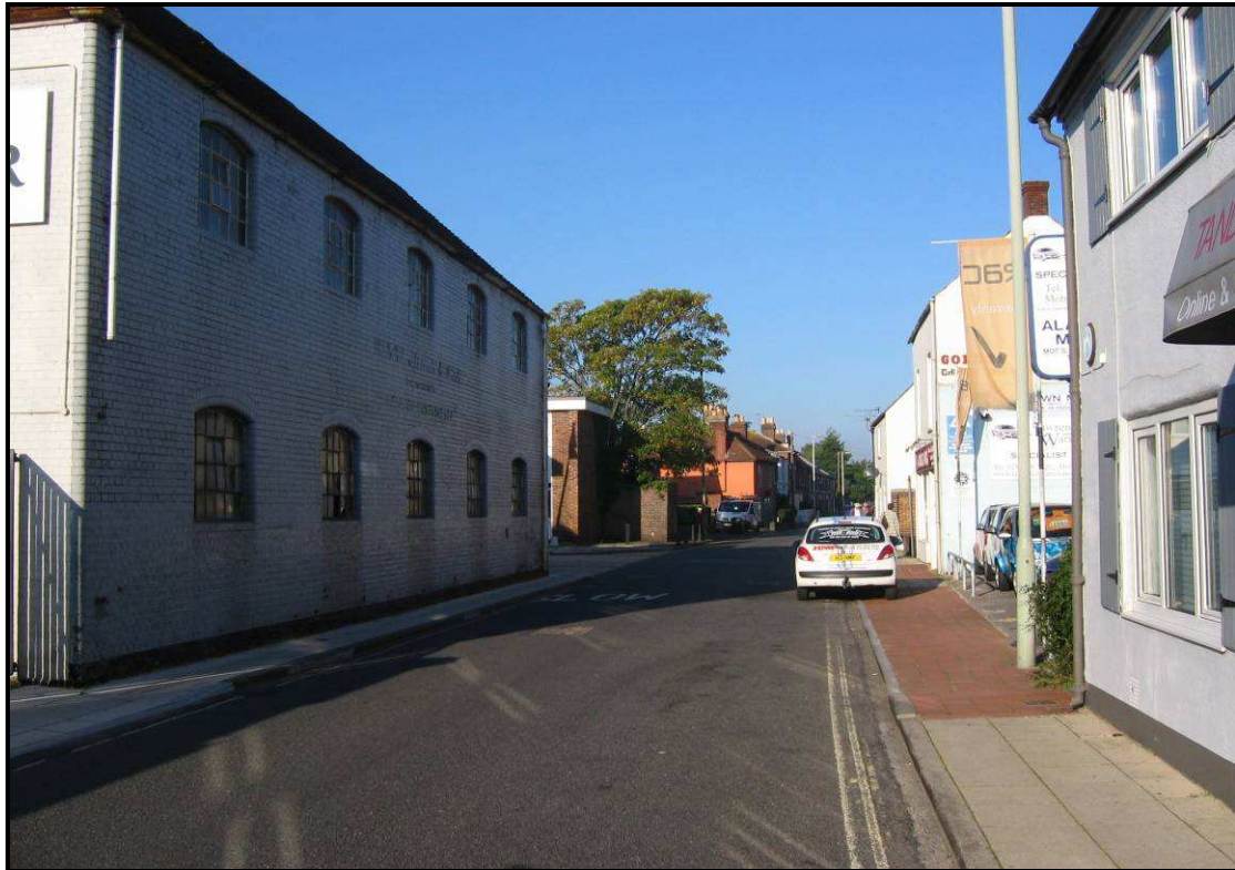
Existing Joinery Building
