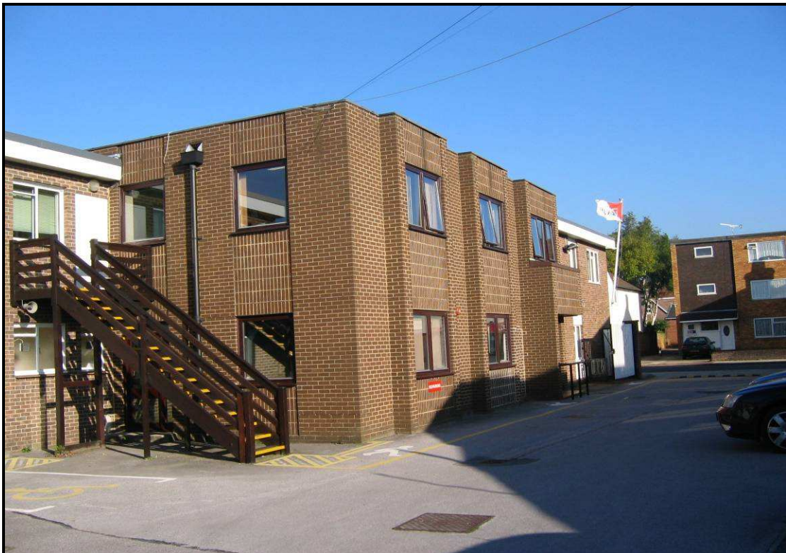
Existing Office Building
