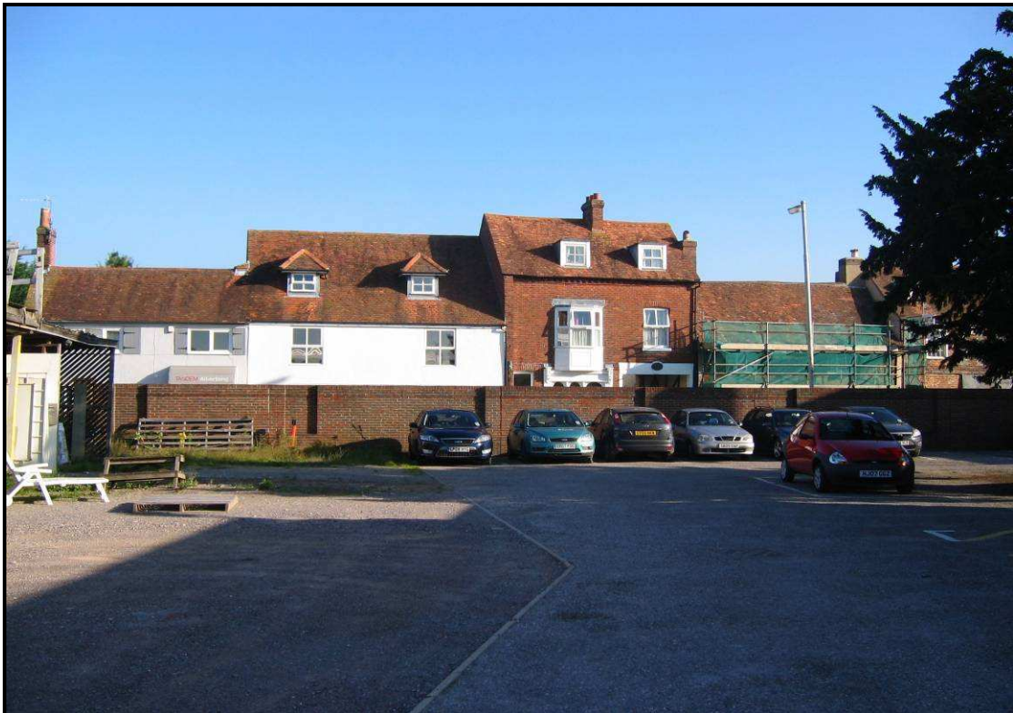
Car Park Wall
