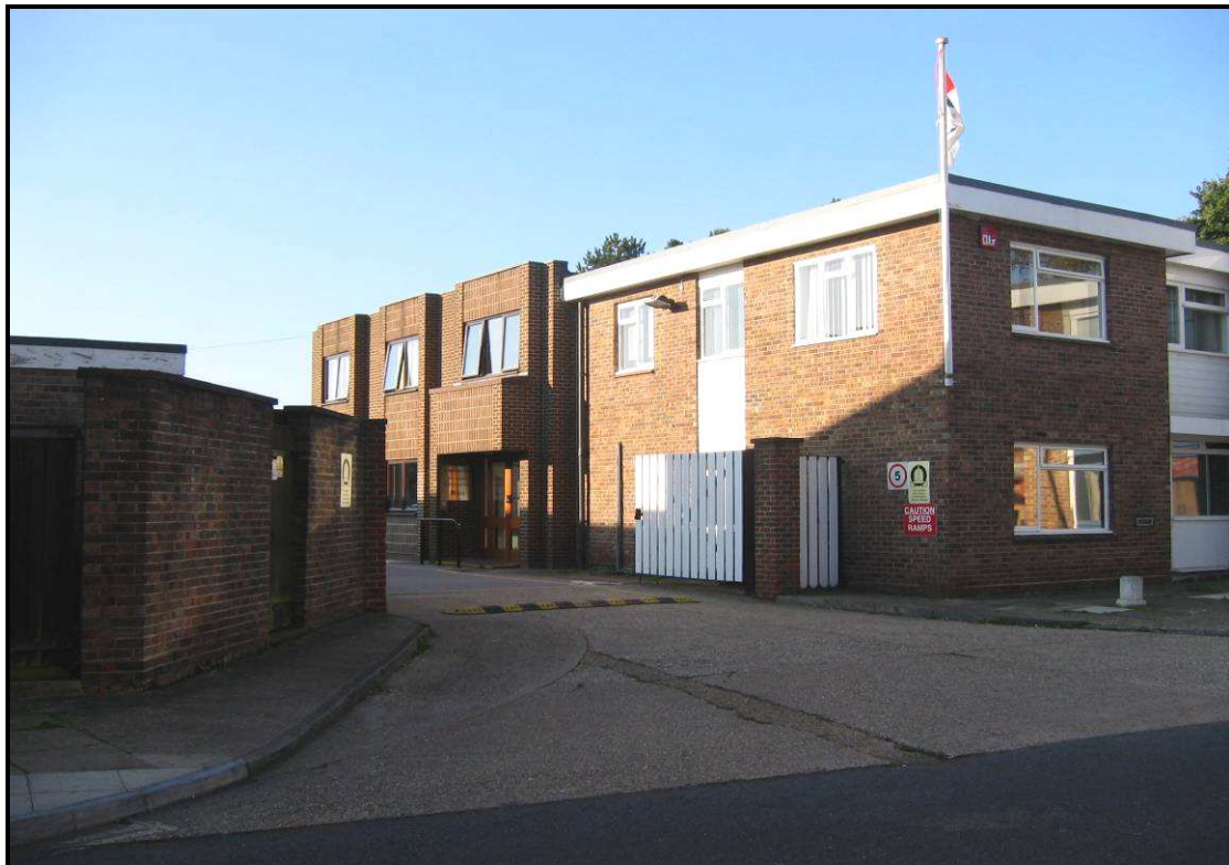
Existing Office Building
