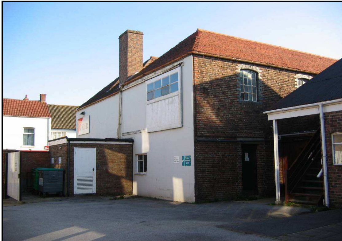
Rear of Joinery Building
