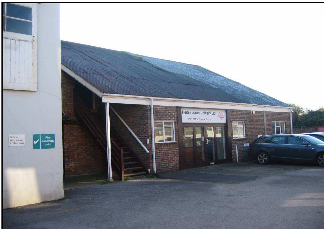
Joinery Building Extension (Rear)
