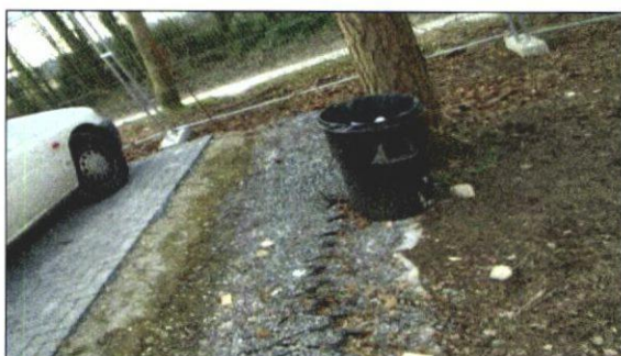
Photo 26: A conventional concrete haunching can be used to retain new surfacing as long as it is not dug into a trench - here it is placed on top of the CellWeb layer.
