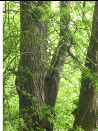
AR15: Vertical crevice with potential to support bats.
