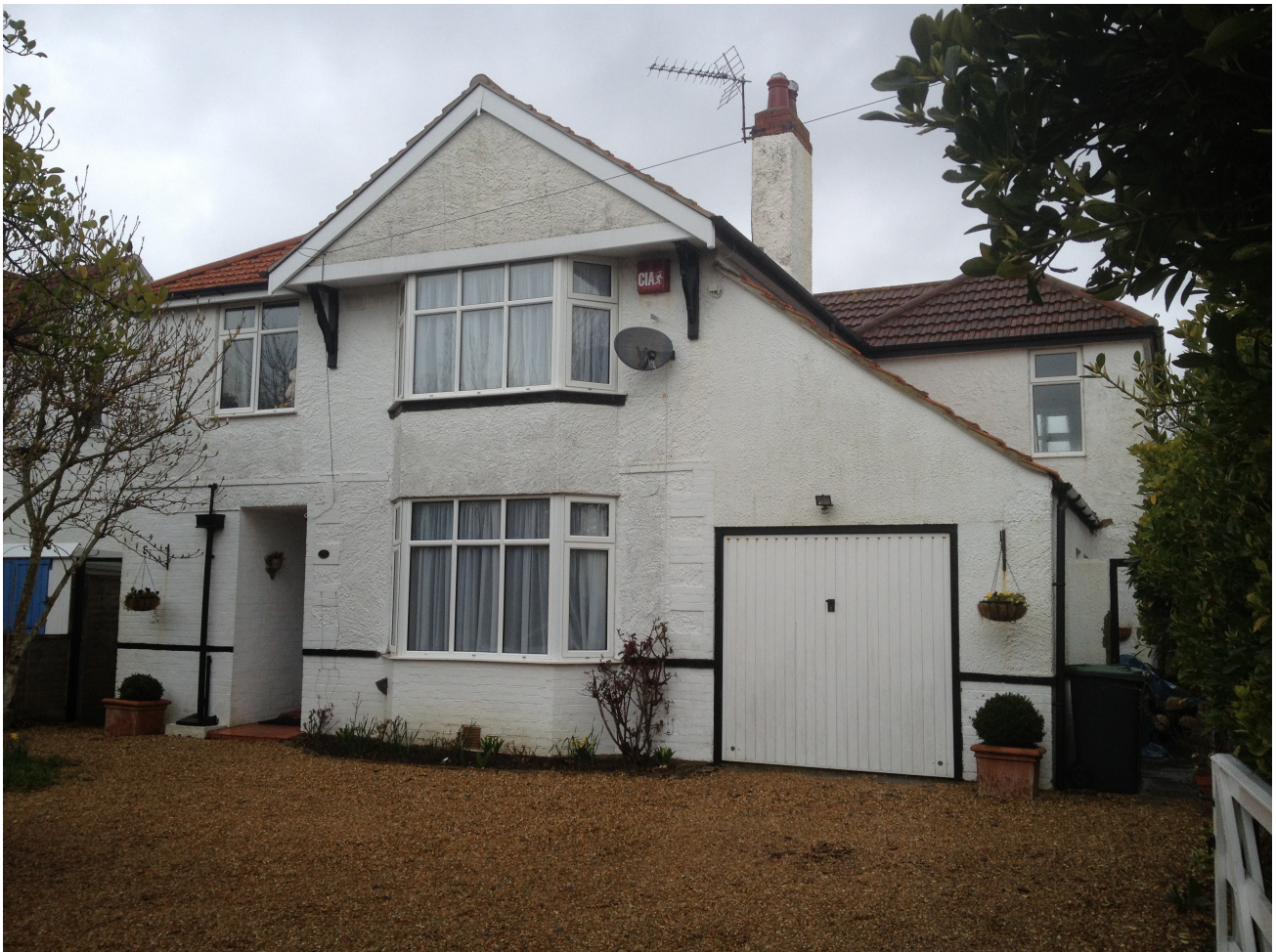
Fig 1. Existing South Elevation
