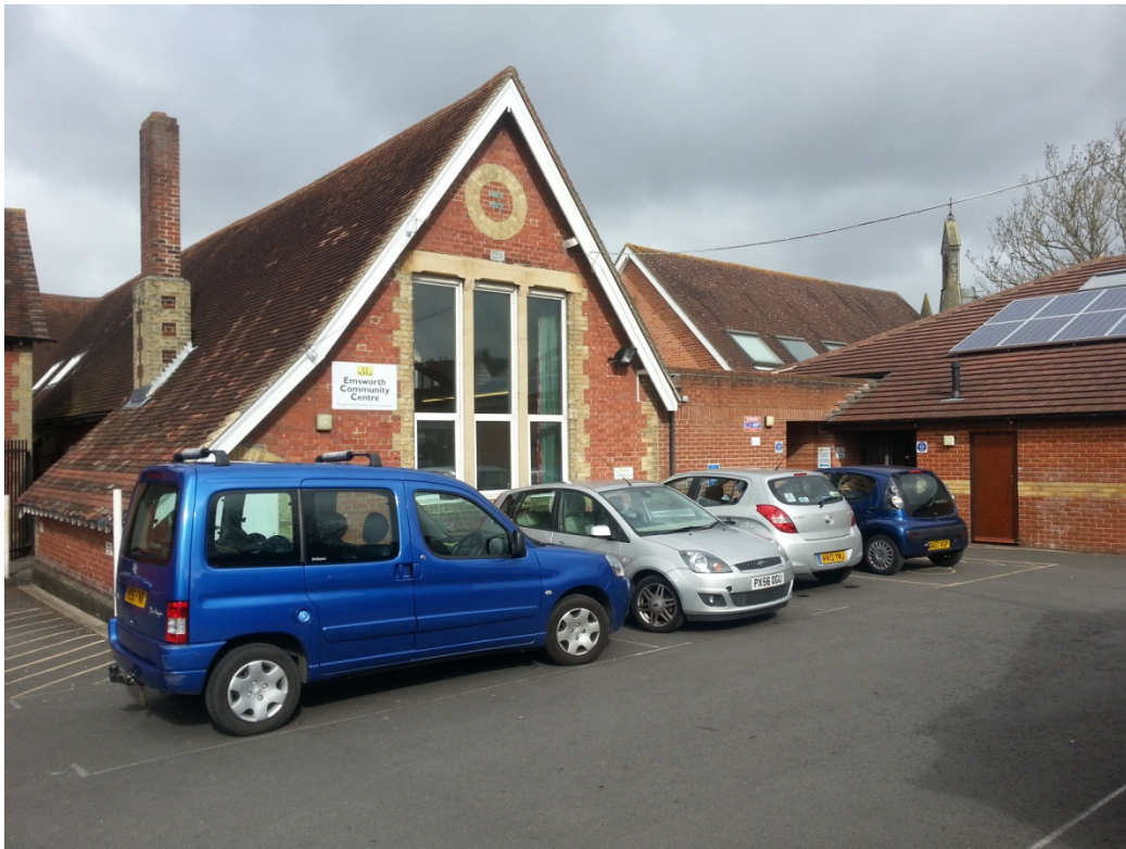
Fig No.1 – Image of Existing Front Elevation & Entrance
