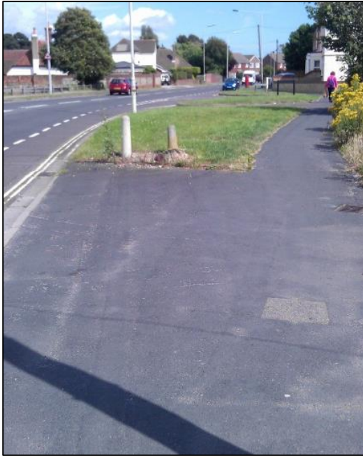
Photograph 2 Footway Fronting the Site
