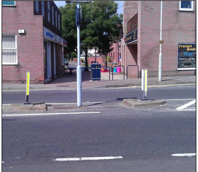
Photograph 3 Existing Traffic Splitter Island & Mengham Shopping Precinct
