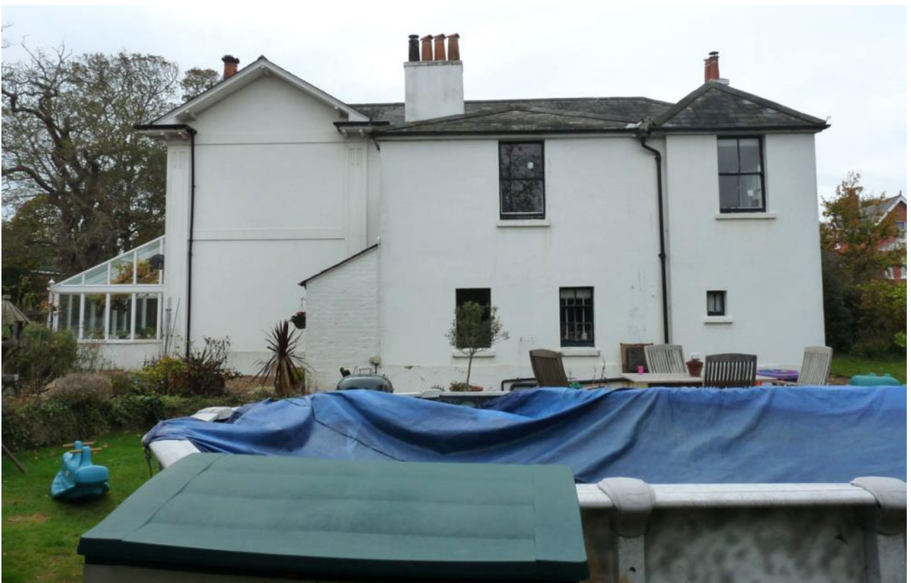
Queensberry Lodge, 15 Hollow Lane, facing North East
