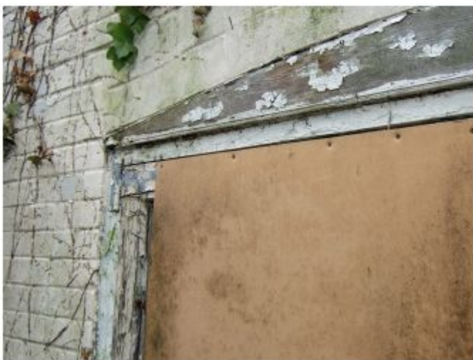
shallow reveal of existing arched doorway to south elevation
