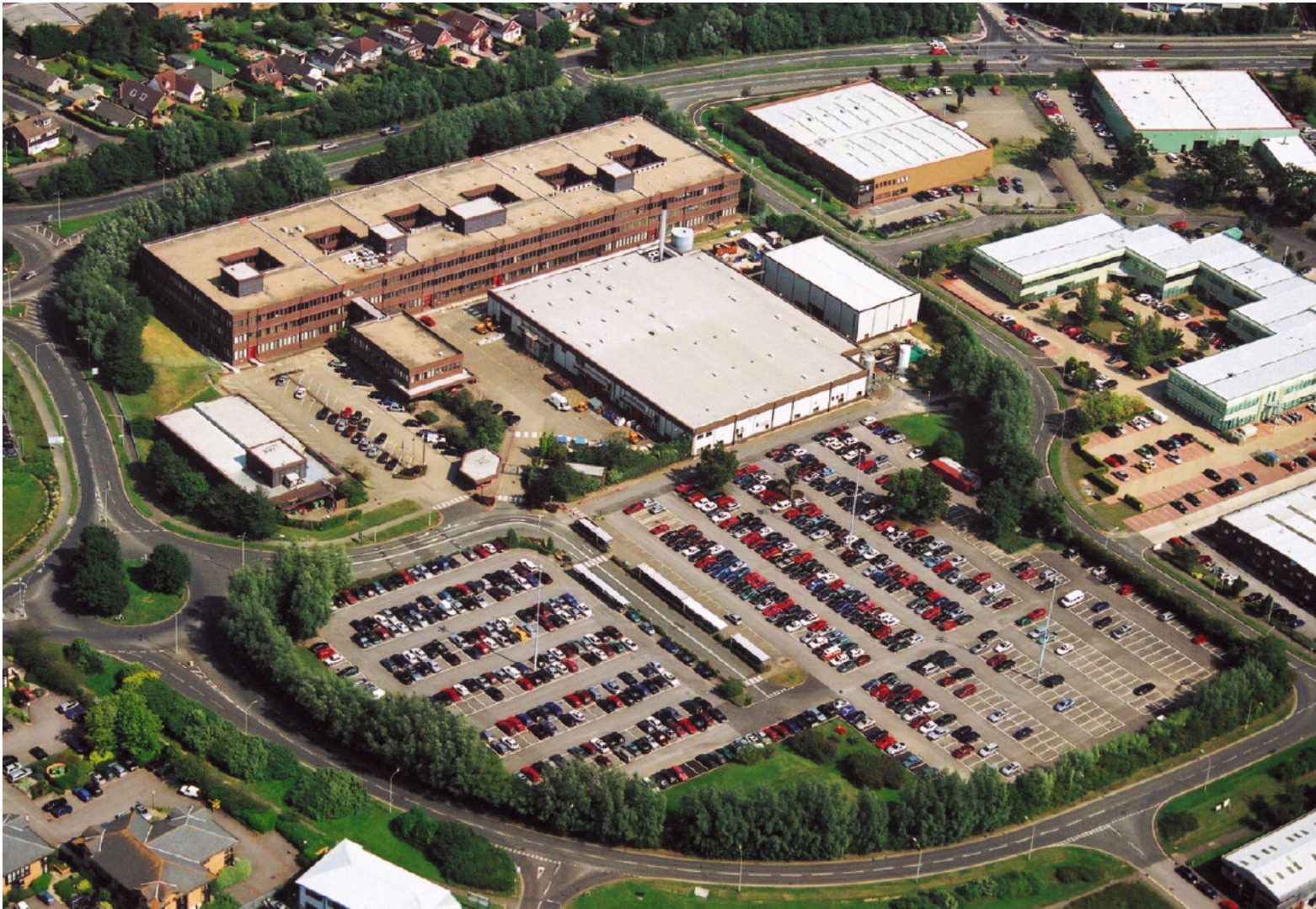
Site aerial from North West corner
