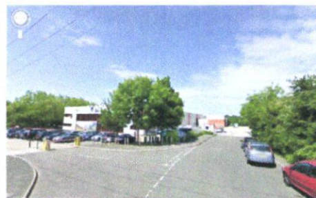
Fig 2: External View of the building.
