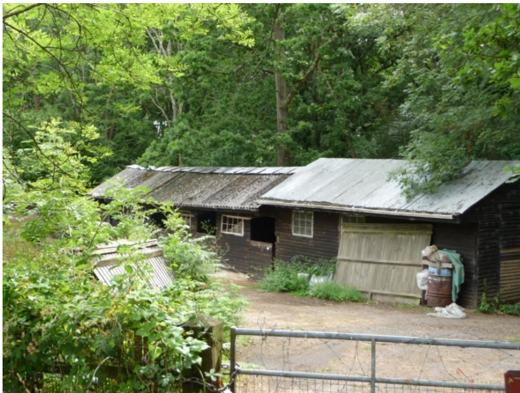
General view of the tenant farmer's barn. The first part of the barn (right-hand side) is made of a corrugated roof with timber boarding as external walls. The second part of the barn (left-hand side) has an asbestos roof with timber boarding as external walls.
