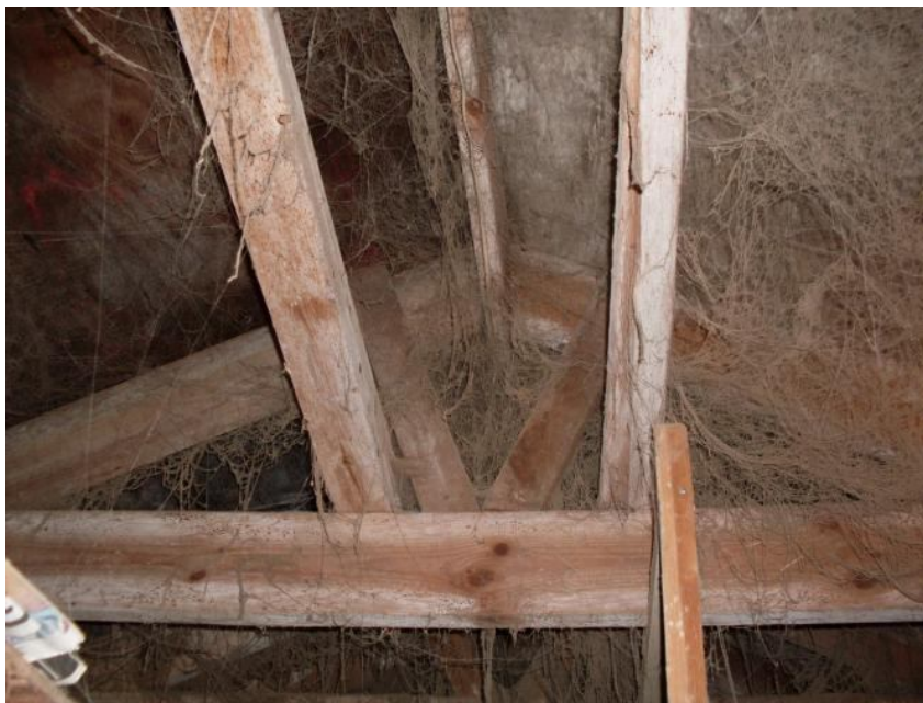
Interior view of the roof from the first section of the barn (with the corrugated roof)
