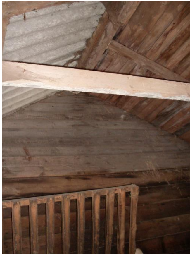
Interior view of the roof from the second section of the barn (with the asbestos roof)
