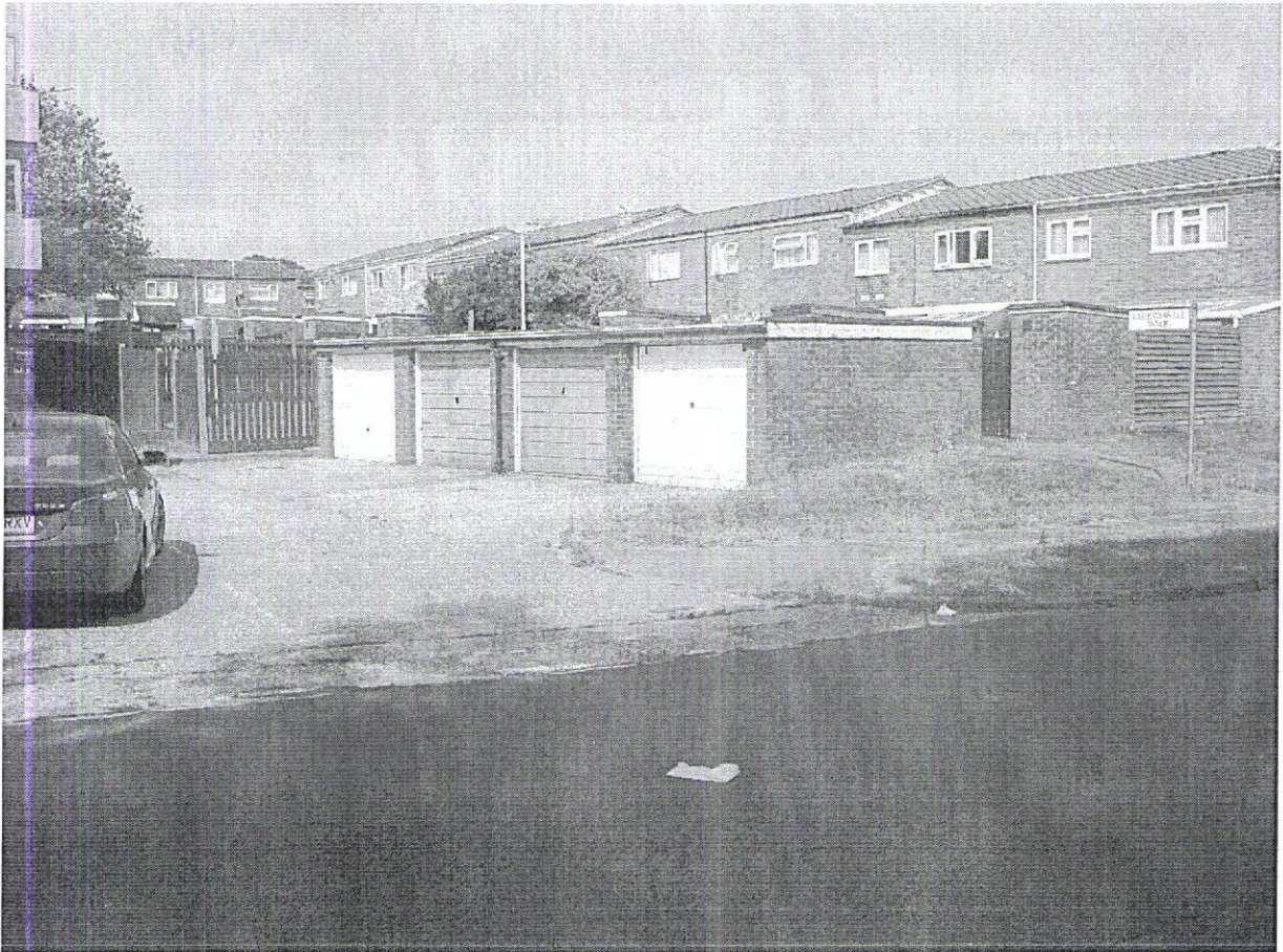
View looking at north western elevation of garages
