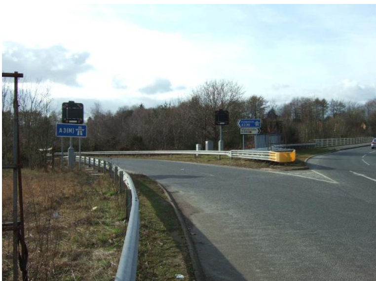
Figure 2. Crash Cushion at A3(M) Junction 3 Southbound On-slip
