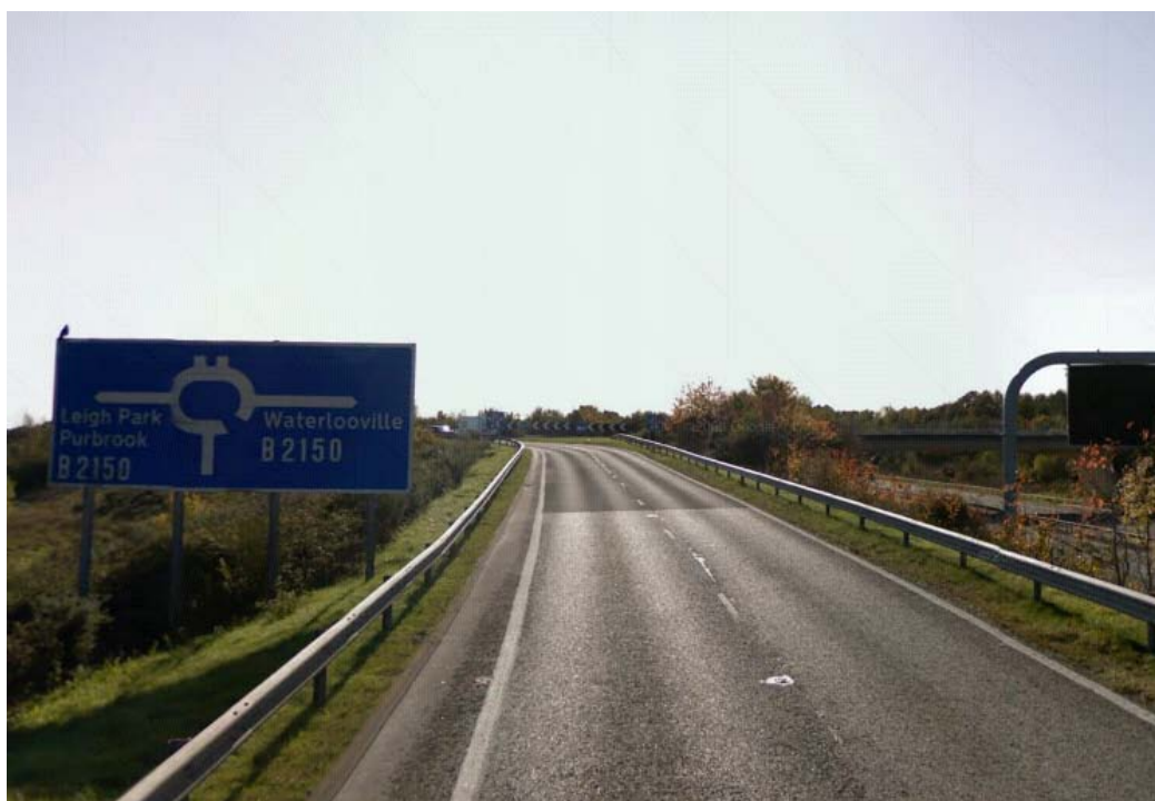
Figure 3.4 – A3(M) Junction 3 – Southbound Off Slip
