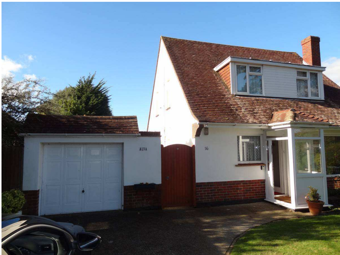
Photo 2 – View of garage and side access with south facing gable to house.
