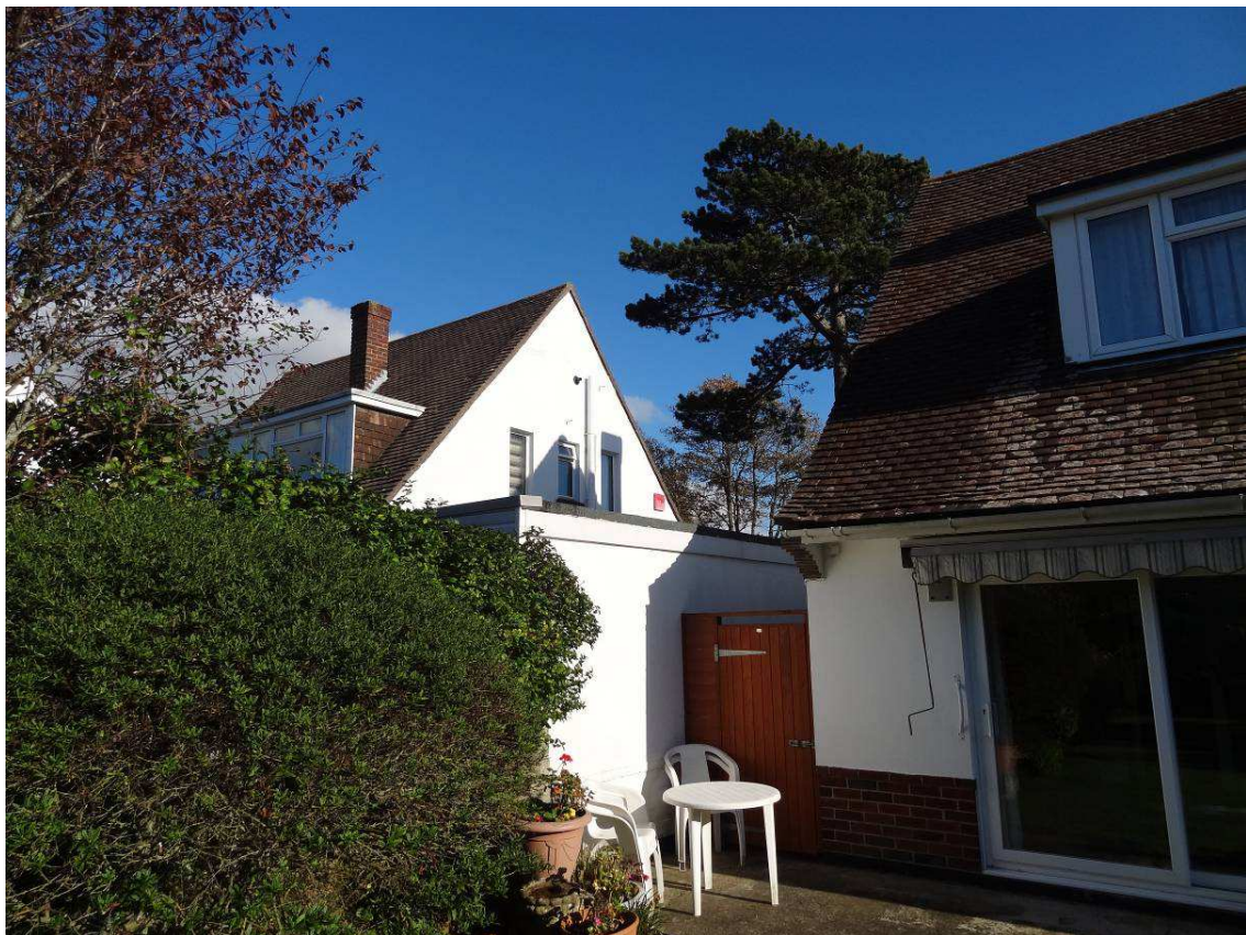
Photo 6 – View looking north-east from garden showing single storey rear addition to adjoining property.
