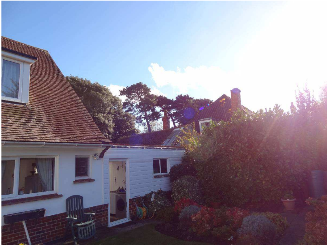
Photo 7 – View looking south-east along from garden showing existing single storey side addition.
