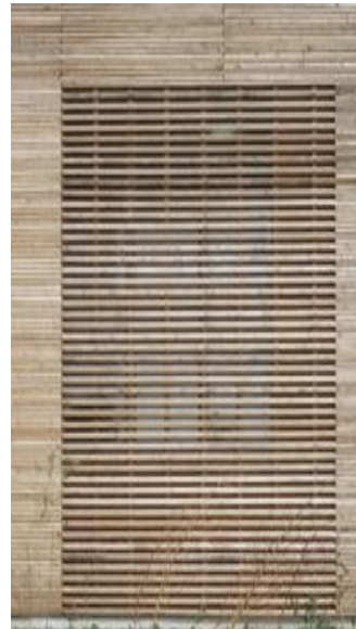
Timber screen with window behind
