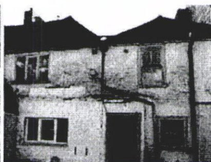
Figure 3 Northern Elevation of Building
