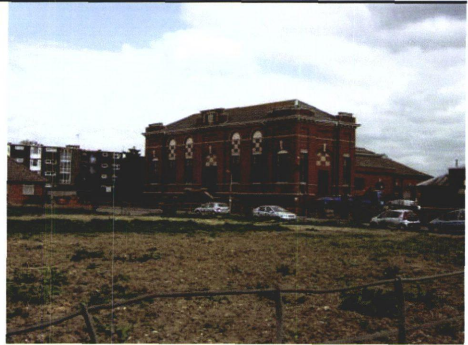
Photo (vi) Significant scale of local industrial heritage – seen from Ranelagh Road looking north east, with four storey flats beyond
