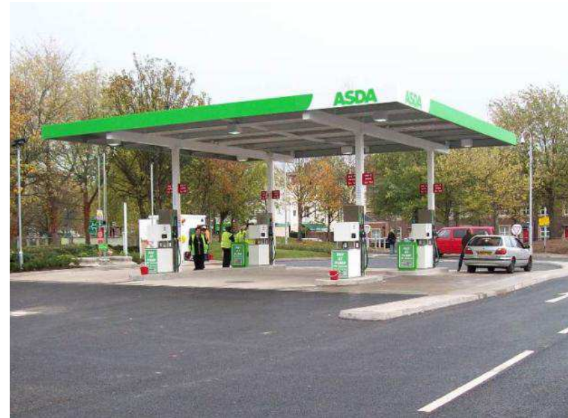
Typical 4 pump PFS Photo
