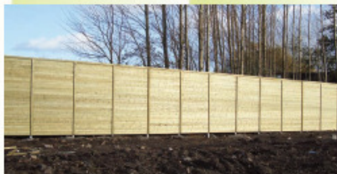
Torwood - 450m of Jakoustic Highway from 4m to 6.5m high
