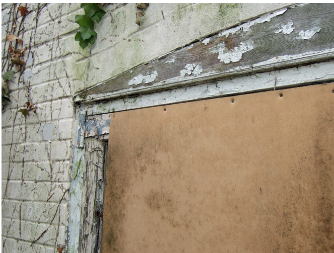
shallow reveal of existing arched doorway to south elevation
