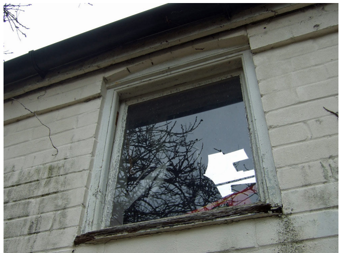
shallow reveal of existing arched window to south elevation
