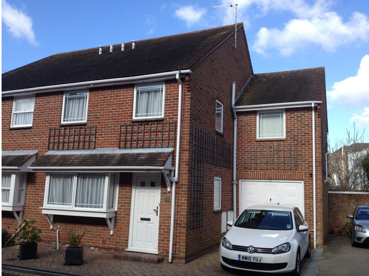
Fig 1: Existing South Elevation
