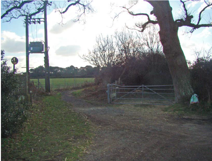
24. View looking south towards public footpath and access to land north of Allocated Site
