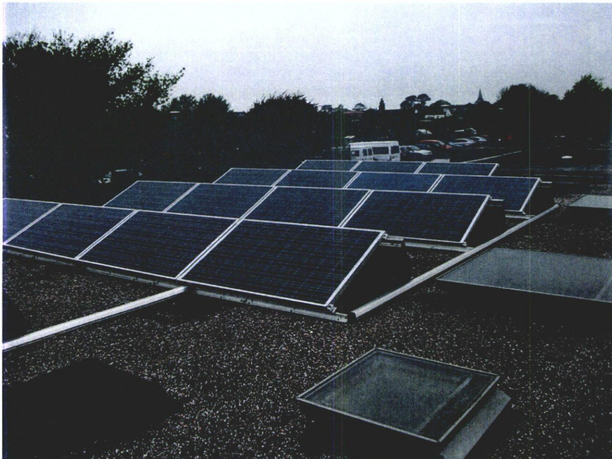
Image 2: Finished installation on the roof of Mengham Junior School
