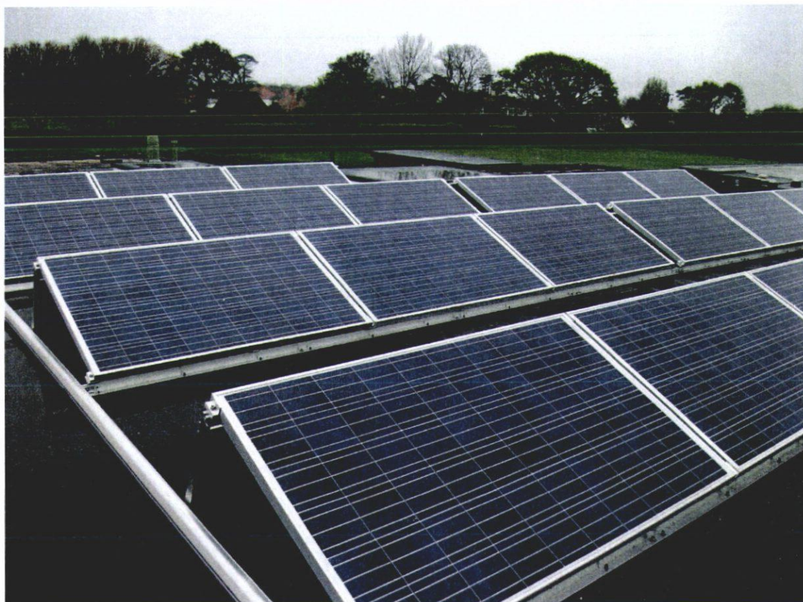
Image 3: Finished installation on the roof of Mengham Junior School
