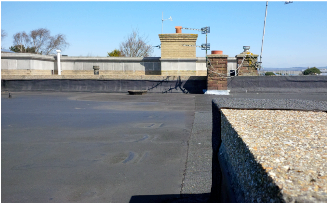
Picture 6 – The bitumen lined flat roof of the No 12 property.
