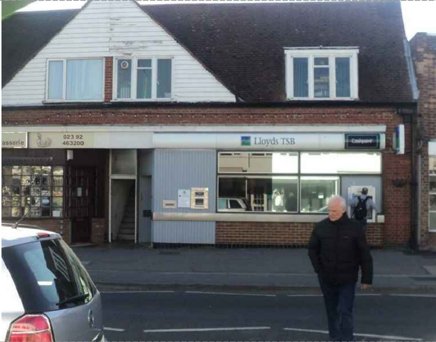
Site Scheme Photo - Existing
