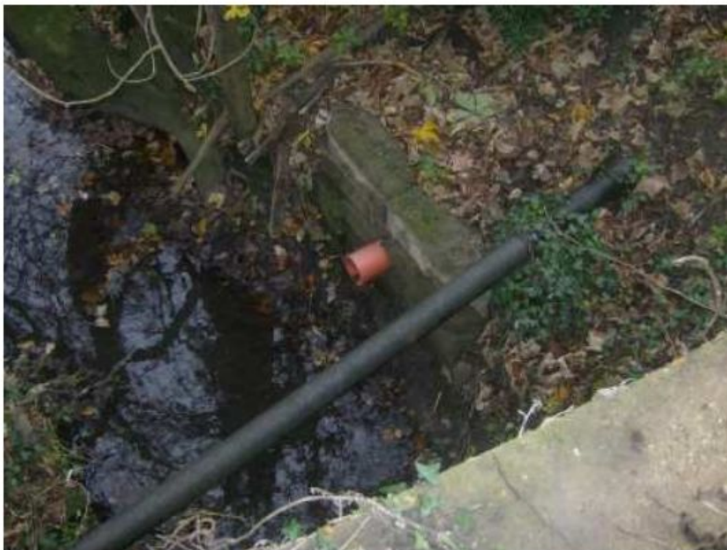
EXISTING STORM OUTFALL TO HERMITAGE STREAM
