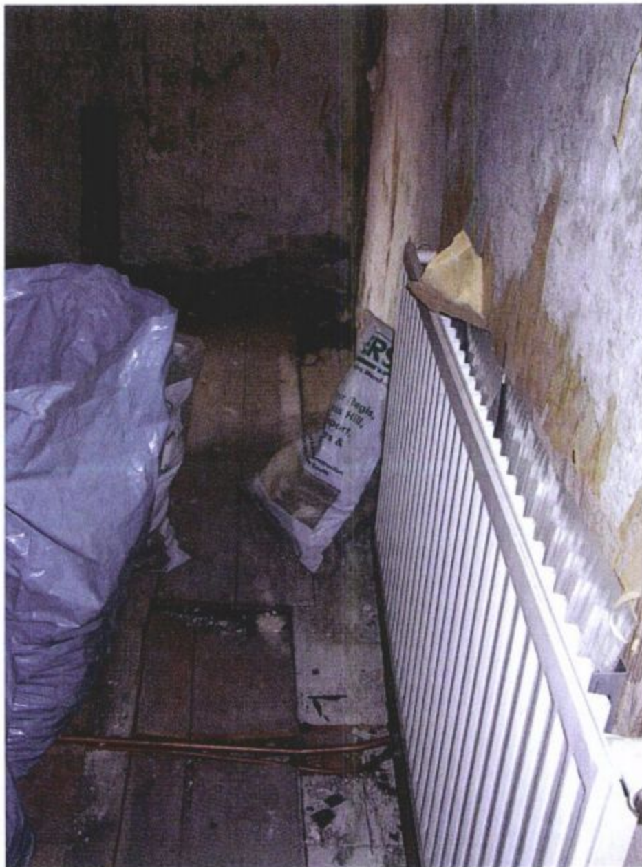
Photo 025 – Corridor. West Party Wall/Bathroom Loadbearing Partition.
