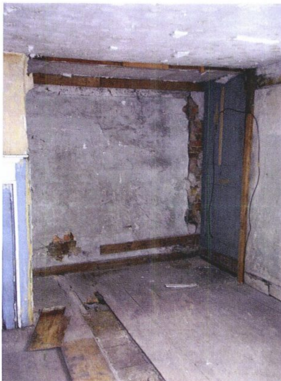
Photo 028 – Bedroom 2. S.E. Corner. Showing East Party Wall.
