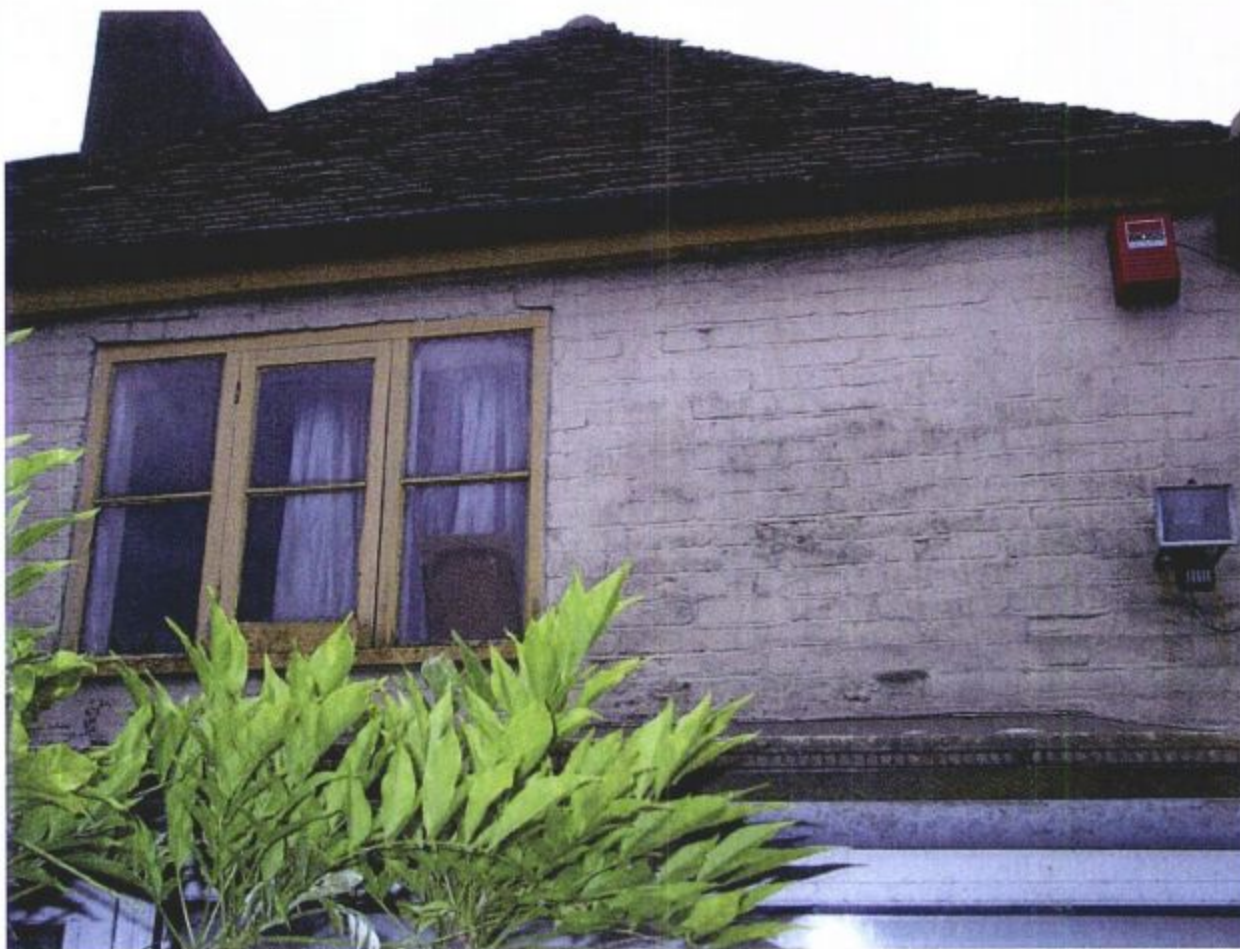
Photo 036 – North Elevation. East Side. N.E. Hip Roof over Bedroom 3.
