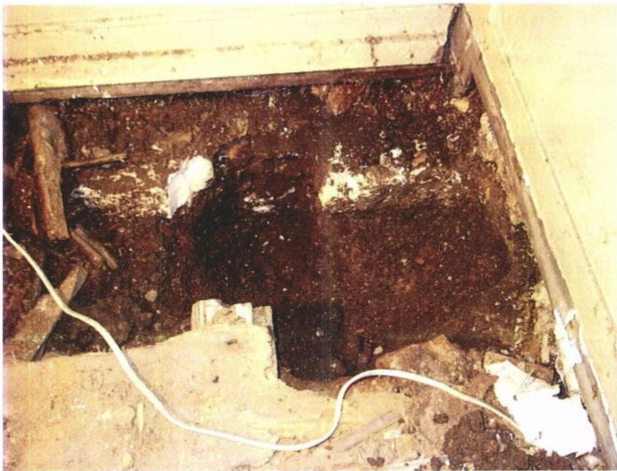
Photo 039 – Lounge. S.E. Corner. Trial Pit Through Timber Ground Floor.
