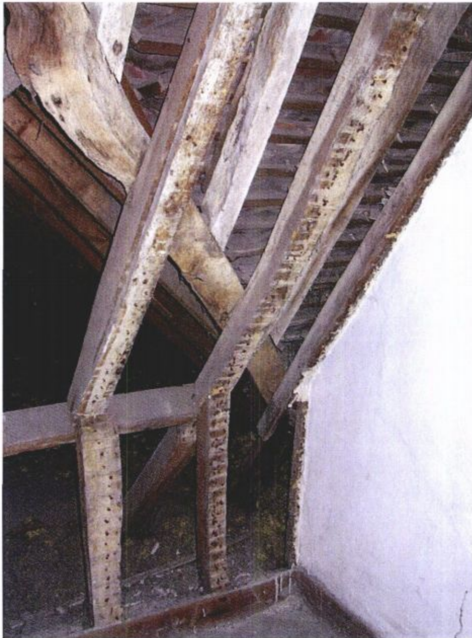
Photo 005 – Roof Accommodation Rear Pitch. Northeast Layboard.
