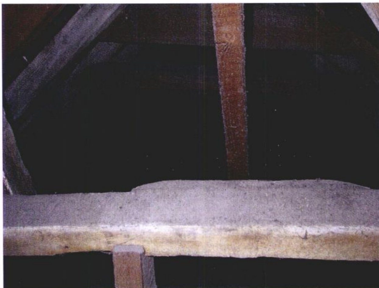
Photo 015 – N.W. Rear Roof Space.
