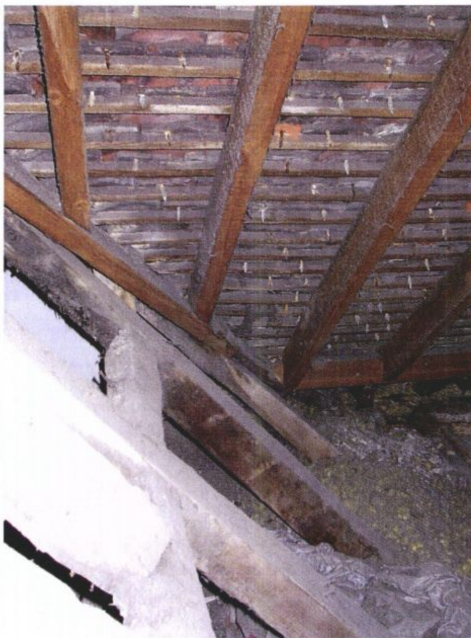
Photo 007 – Rear West Pitch behind Roof Accommodation Area.
