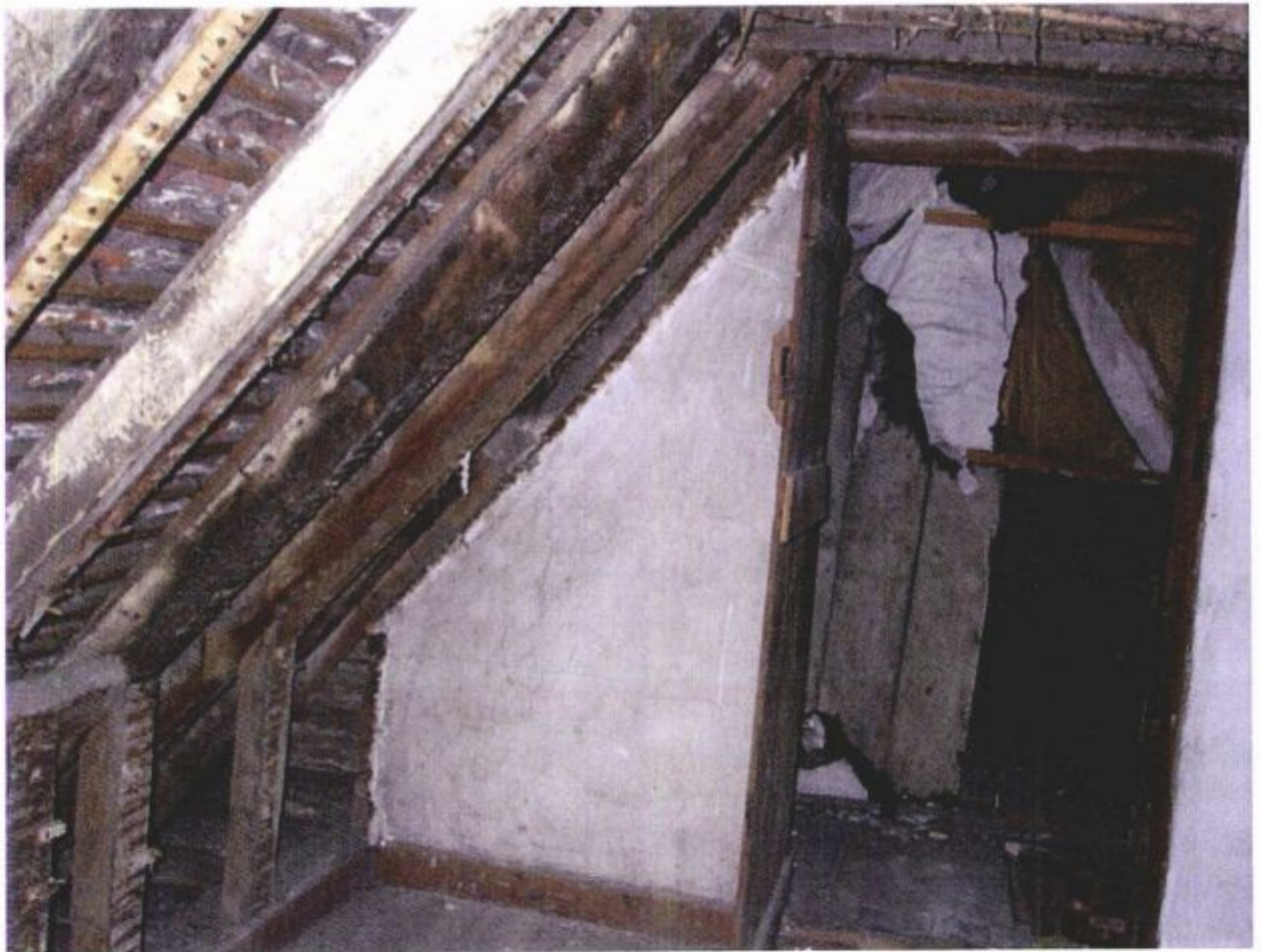
Photo 010 – Roof Accommodation Area. S.W. Corner, Front Pitch.
