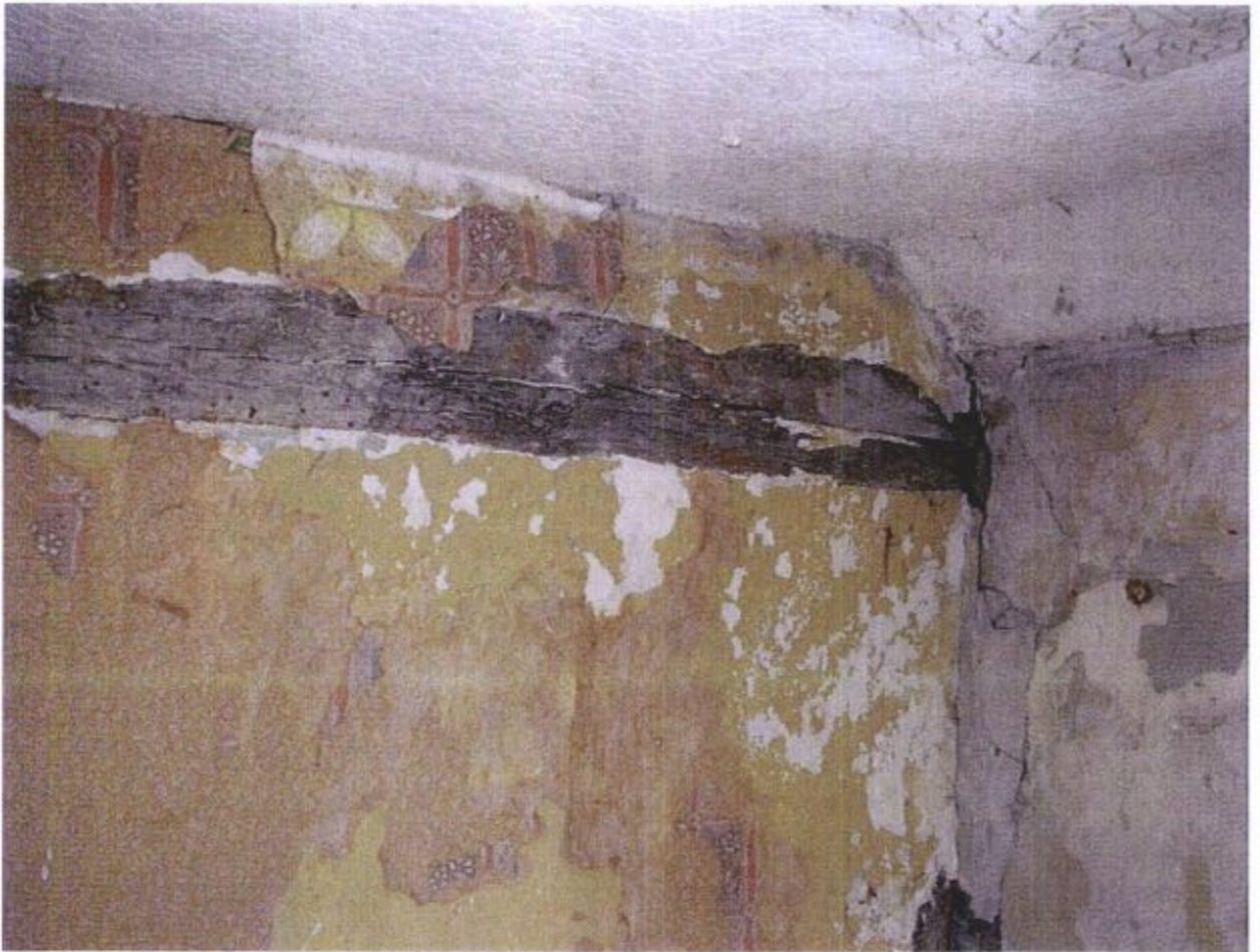
Photo 021 – Bedroom 1. S.E. Corner. Partition Junction with South Wall at Frame Head.
