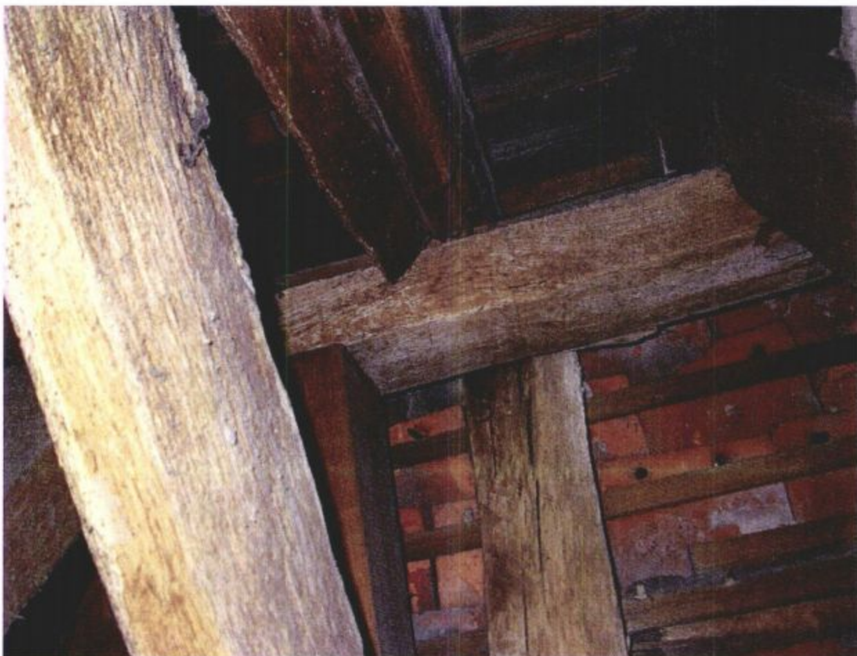
Photo 016 – Front S.W. Roof Space. Ridge Beam Adjacent Stair.
