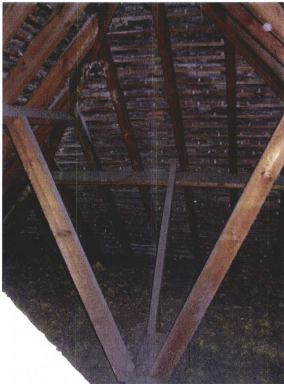
Photo 006 – E-W Roof behind Roof Accommodation Area.
