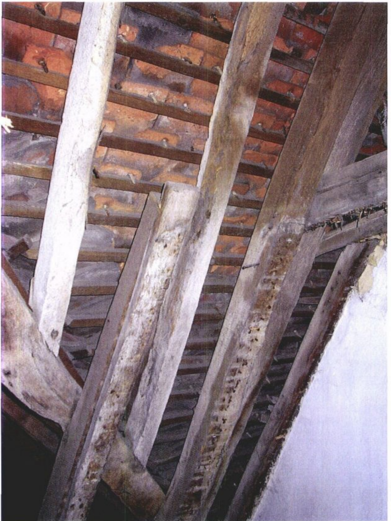
Photo 004 – Roof Accommodation Area. Rear Pitch Northeast Layboard/Beam.
