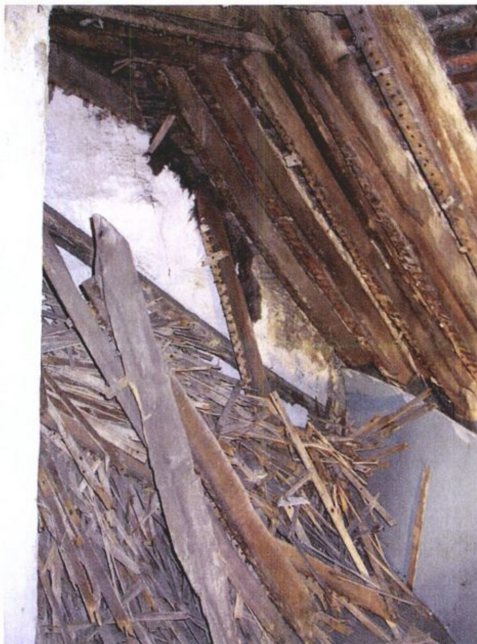
Photo 002 – East Party Wall in Roof Adjacent Stack.
