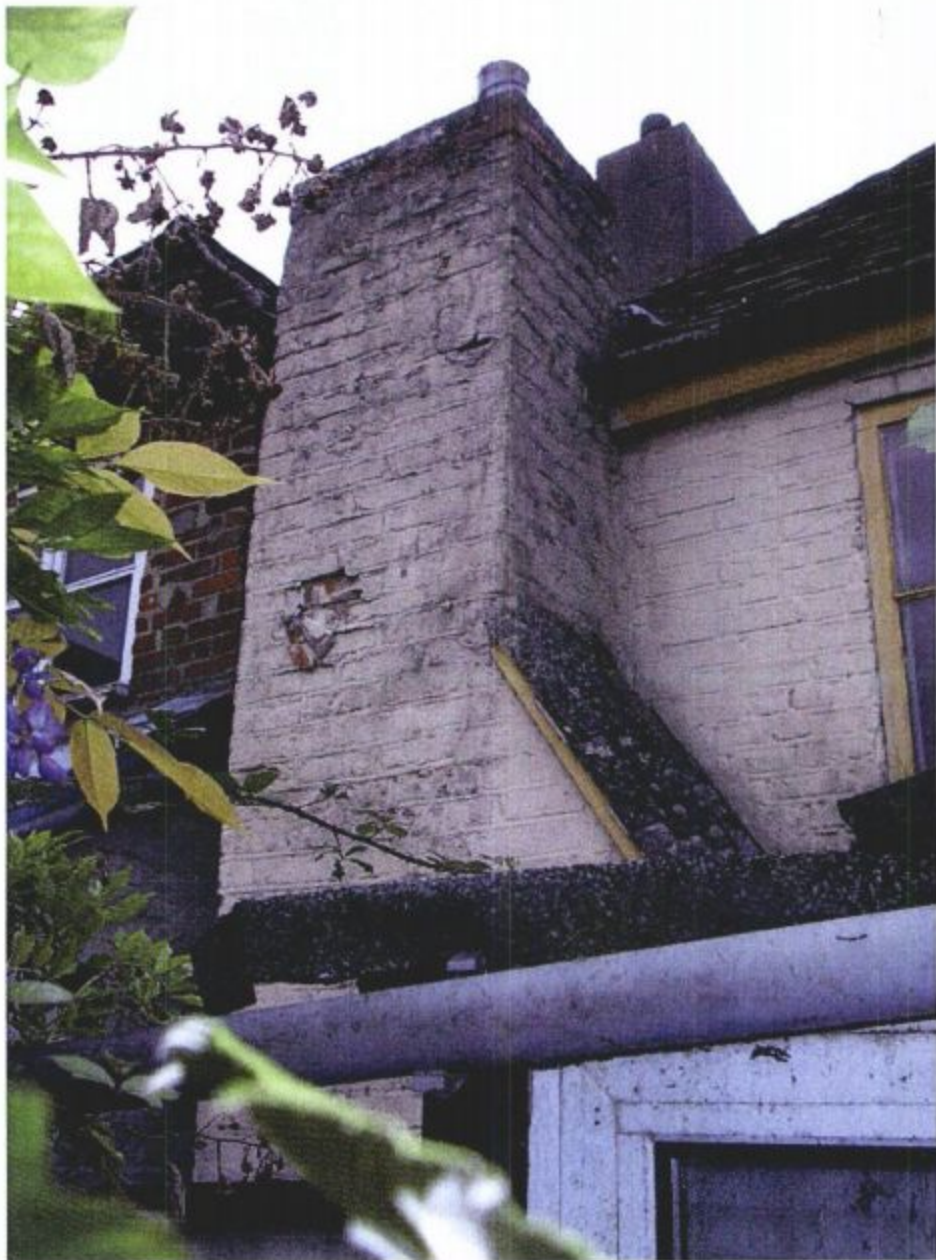
Photo 037 – North Elevation. N.E. Corner Stack.
