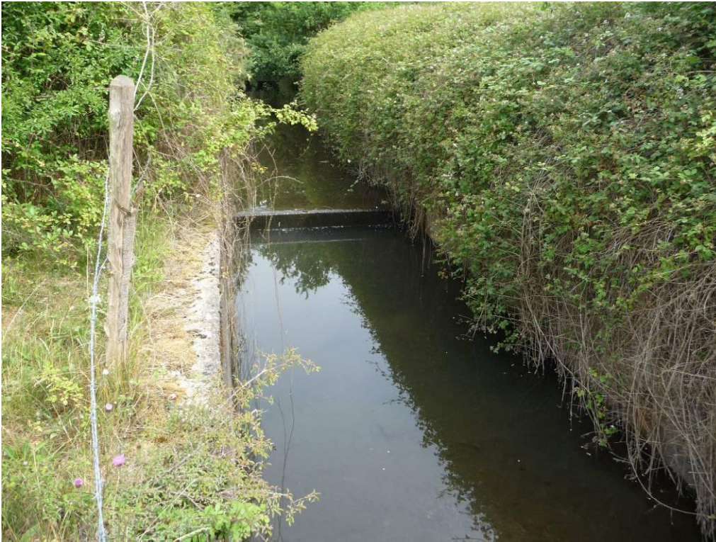
Photograph 5. Hermitage Stream showing bramble scrub at proposed link road crossing bridge location (Listening station no 8). (Photograph taken from walkover survey in 2011 and habitats have not changed prior to transect survey in 2012).
