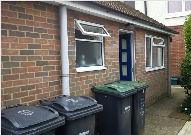
EXISTING REAR EXTENSION (showing front door to bedsit)
