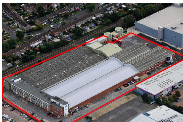
View of the site
