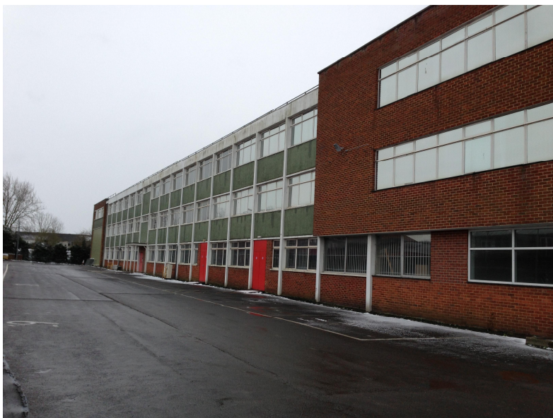
Existing redundant offices on north elevation
