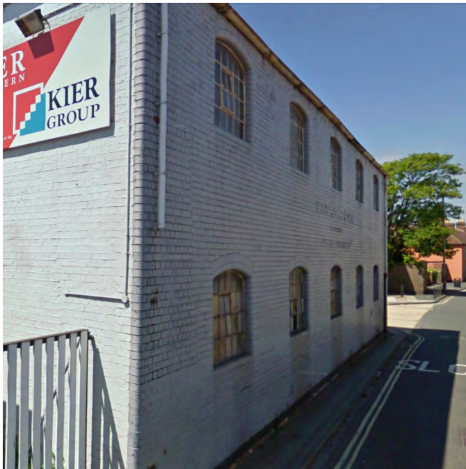
View 8 – Existing building along West Street to be retained
