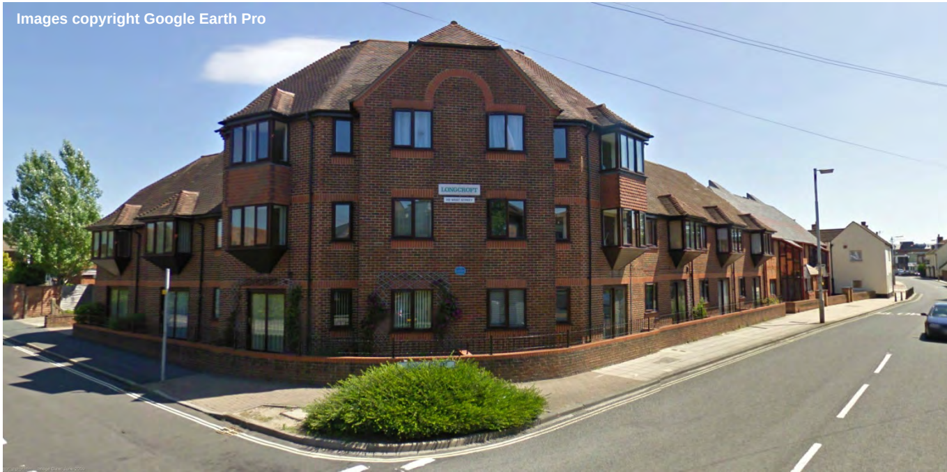
View 1 – Corner building on West Street / Boundary Way junction
