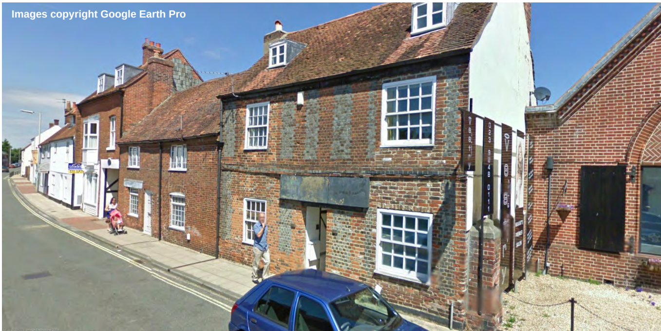
View 4 – Terraced units along West Street opposite site
