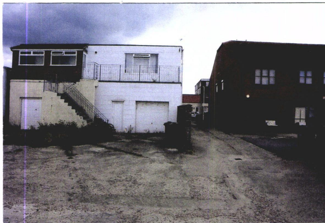
Rear elevation of Nos. 29/29A, Creek Road from car parking area.
