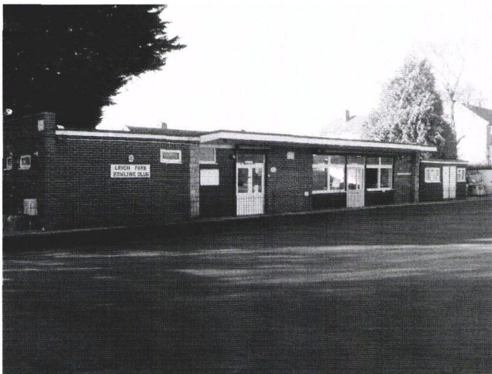
East (front) view of the club house with the previous detached changing rooms on the far right hand side.
