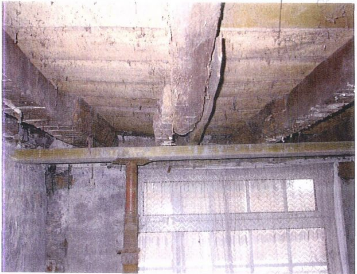
Photo No. 51 – Study:- 1 st Floor Joists.
